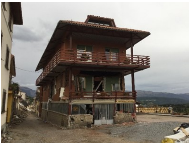
Fig. 1: A typical existing steel frame in the municipality of Amatrice, Central Italy, which was damaged during the 2016-2017 Central Italy earthquake sequence
