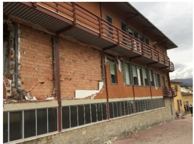
Fig. 1: A typical existing steel frame in the municipality of Amatrice, Central Italy, which was damaged during the 2016-2017 Central Italy earthquake sequence
